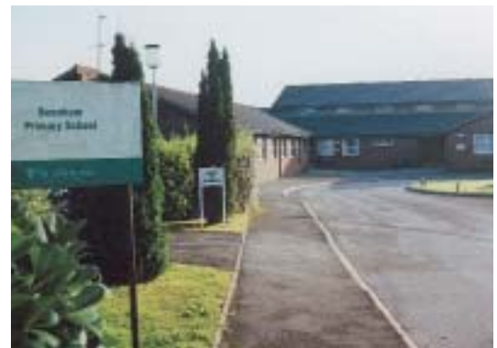
In a village with decreasing facilities the school plays a pivotal role, socially and physically, with the community room under the same roof
